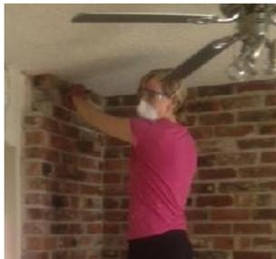
Gloves, protective eye wear, face mask and clothes suitable for hard work and wear-and-tear are all on the 'best dressed list' for anyone doing hands-on DIY work.
